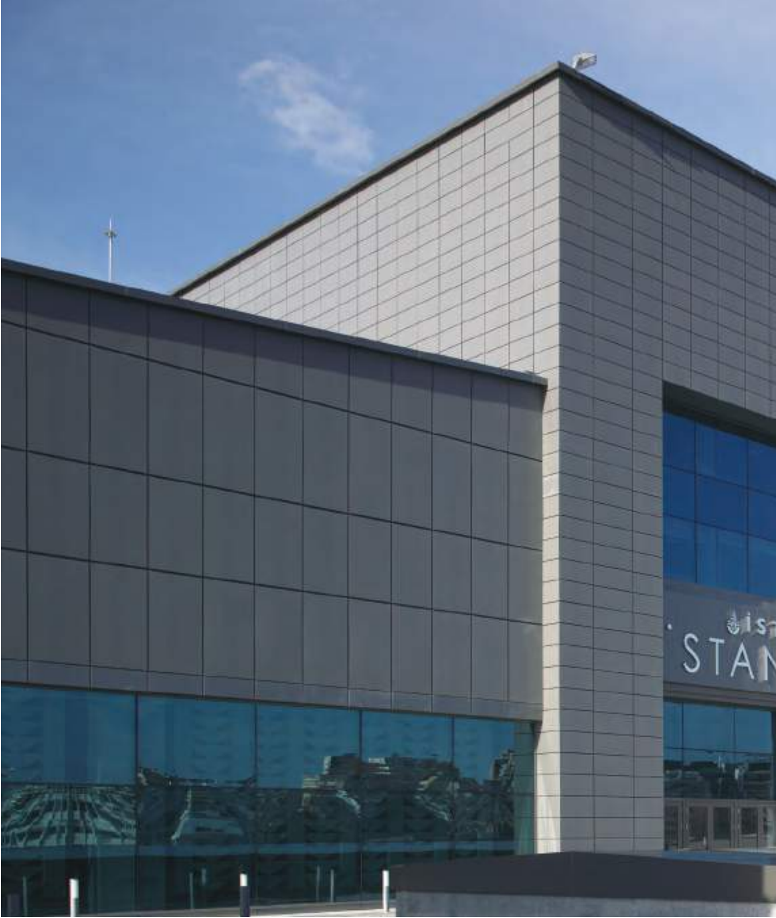
Lütfi Kırdar Kongre Merkezi / İstanbul — Kalesinterflex 3mm Fit Mat Özel Renk / Gizli Klipsli Sistem Lütfi Kırdar Convention Center / İstanbul — Kalesinterflex 3mm Fit Matte Special Color / Hidden Clips Fitted Facade System Mimar: Arima Mimarlık — Architect: Arima Architectural Office
