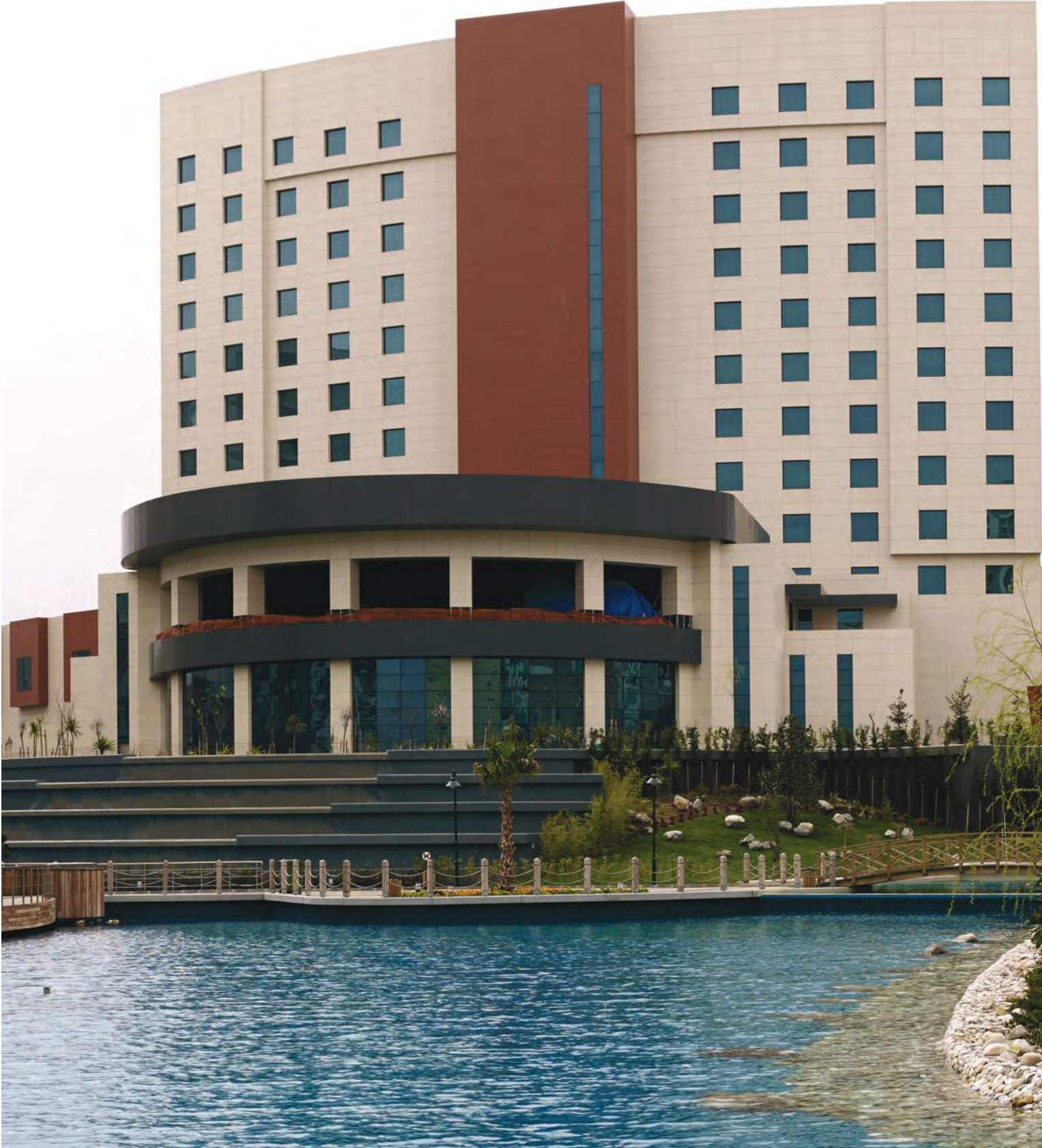
Avrupa Konutları Acıbadem Atakent Hastanesi, Halkalı / İstanbul — Kalesinterflex 3mm Fit Mat Beyaz, Kalesinterflex 3mm Fit Mat Kızıl / Gizli Klipsli Sistem Avrupa Residence Acıbadem Atakent Hospital, Halkalı / İstanbul — Kalesinterflex 3mm Fit Matte White, Kalesinterflex 3mm Fit Matte Coral / Hidden Clips Fitted Facade System Mimar: Arta Mimarlık — Architect: Arta Architectural
