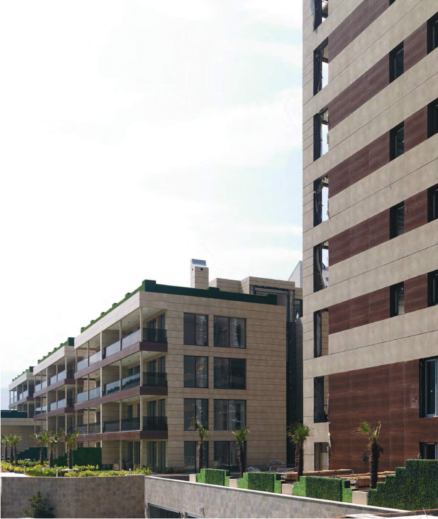
Misia Konutları, Bursa / Kalesinterflex 3mm Fit Luxury Cement Fildişi, 3mm Fit Technowood Ceviz / Gizli Klipsli Sistem Misia Residence, Bursa / Kalesinterflex 3mm Fit Luxury Cement Ivory, 3mm Fit Technowood Walnut / Hidden Clips Fitted Facade System Mimar: Emre Arolat Architects — Architect: Emre Arolat Architects
