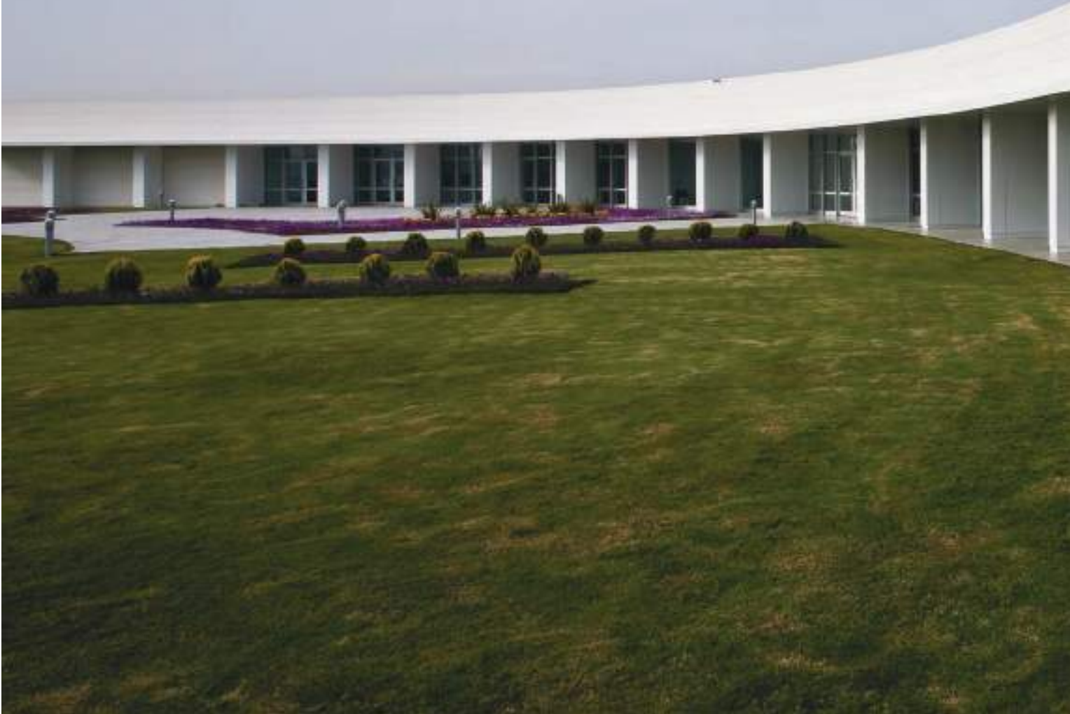
İTOB Yönetim Binası, Menderes / İzmir — Kalesinterflex 3mm Fit Mat Beyaz / Gizli Klipsli Sistem İTOB Administration Building, Menderes / İzmir — Kalesinterflex 3mm Fit Matte White / Hidden Clips Fitted Facade System Mimar: Pao Mimarlık — Architect: Pao Architectural Office
