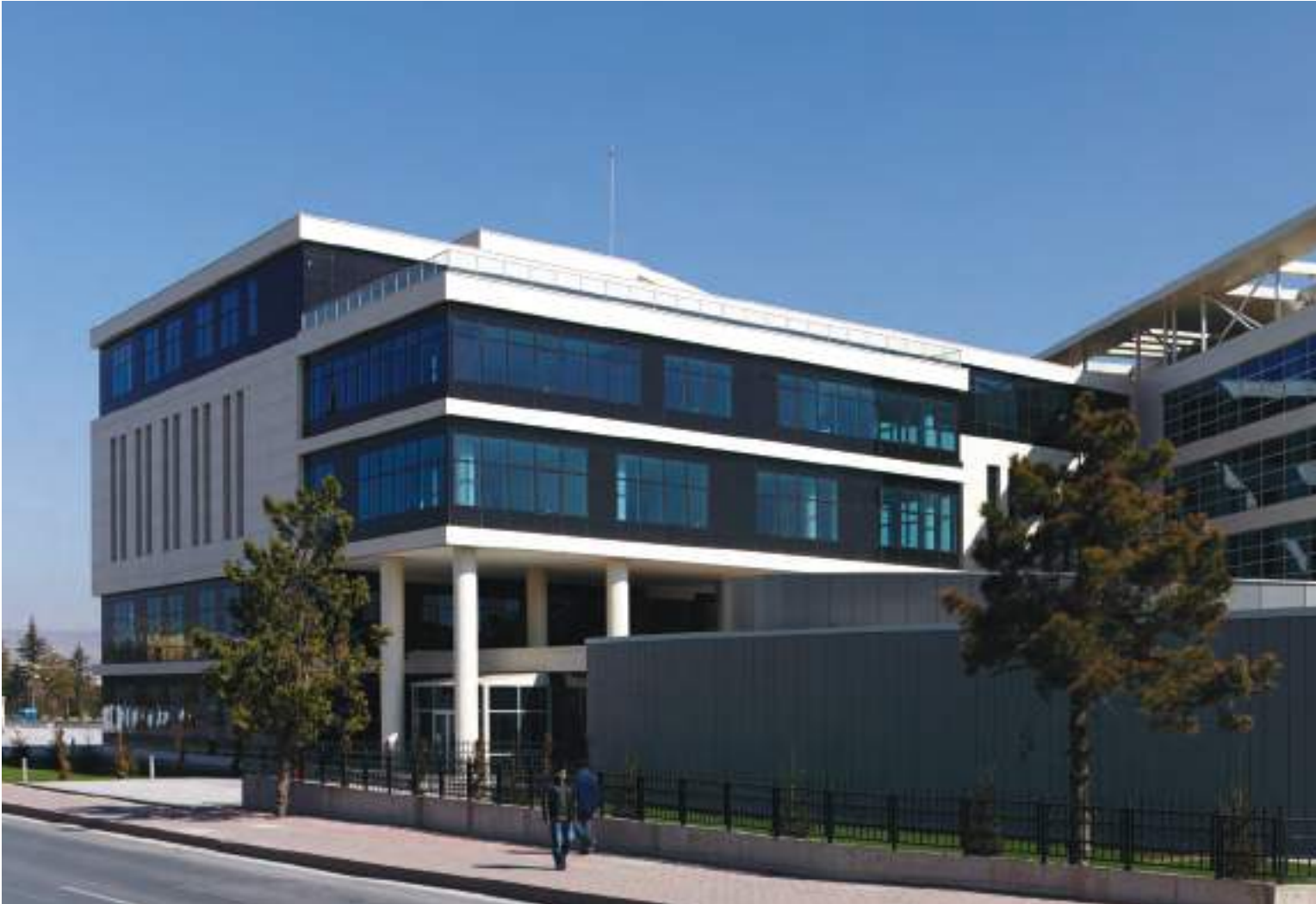
Kayseri Adliye Sarayı / Kayseri — Kalesinterflex 3mm Fit Mat Beyaz, 3mm Fit Mat Çimento Gri, 3mm Fit Mat Fildişi / Gizli Klipsli Sistem Kayseri Courthouse / Kayseri — Kalesinterflex 3mm Fit Matte White, 3mm Fit Matte Cement Grey, 3mm Fit Matte Ivory / Hidden Clips Fitted Facade System Mimar: Ven Mimarlık — Architect: Ven Architects
