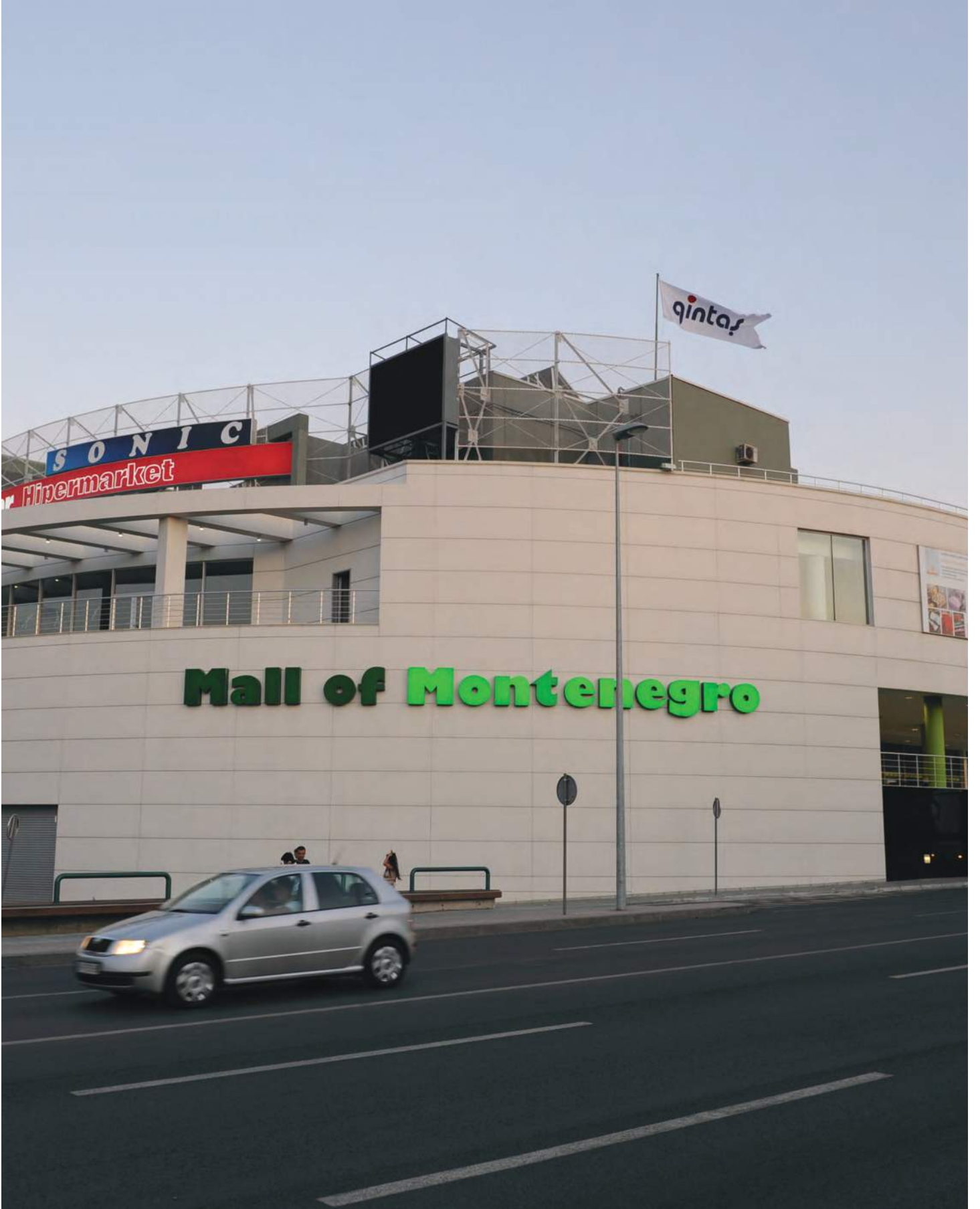
Montenegro AVM / Karadağ — Kalesinterflex 3mm Fit Mat Beyaz / Gizli Klipsli Sistem Montenegro AVM / Karadağ — Kalesinterflex 3mm Fit Matte White / Hidden Clips Fitted Facade System Mimar: Mars Mimarlar — Architect: Mars Architects
