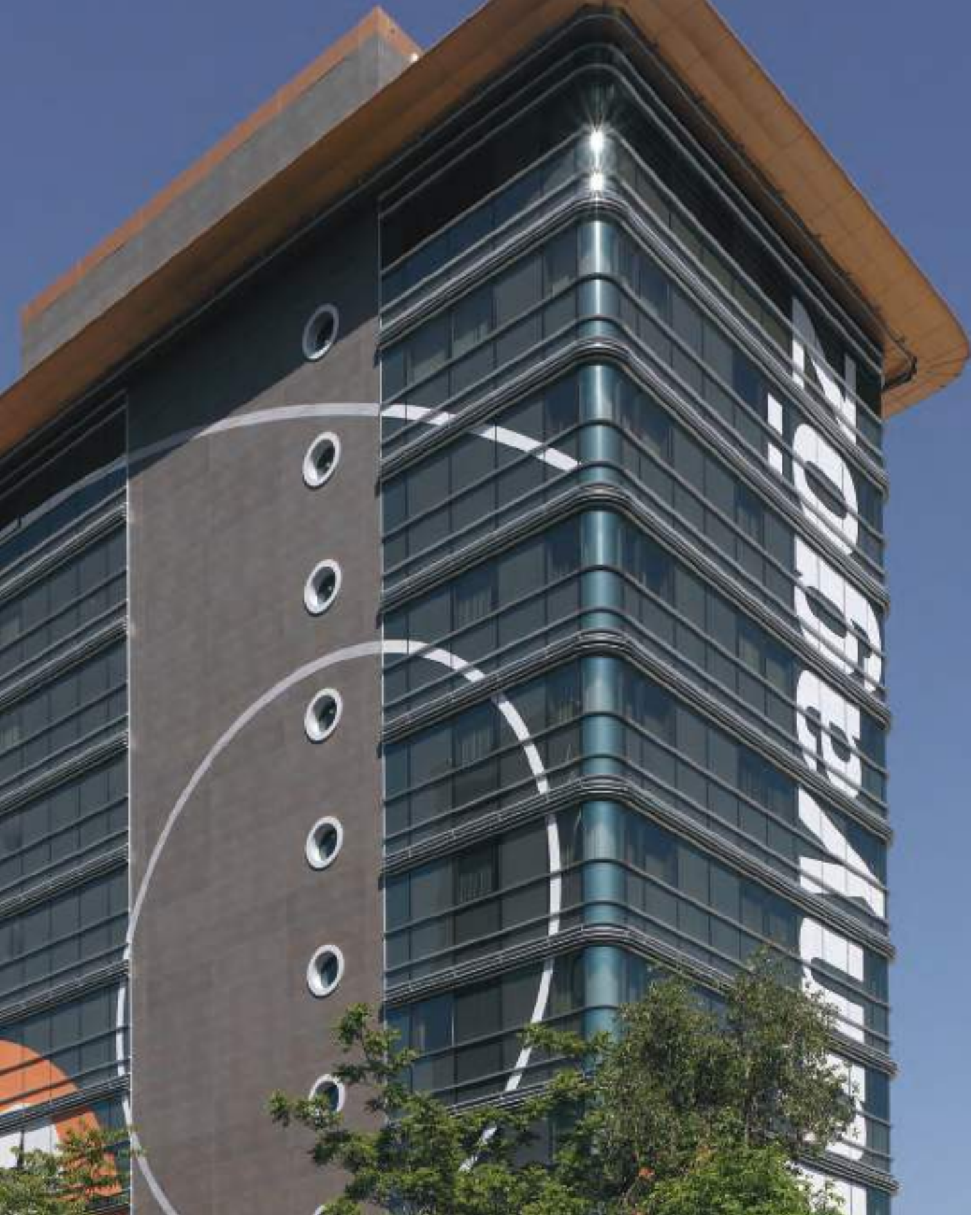
Dnyaya Gz Hastanesi / Ankara — Kalesinterflex 3mm Fit Luxury Cement Vizon / Gizli Klipsli Sistem Dnyaya Gz Hospital / Ankara — Kalesinterflex 3mm Fit Luxury Cement Mink / Hidden Clips Fitted Facade System Mimar: Ahmet Öztürk Mimarlık — Architect: Ahmet Öztürk Architectural Office
