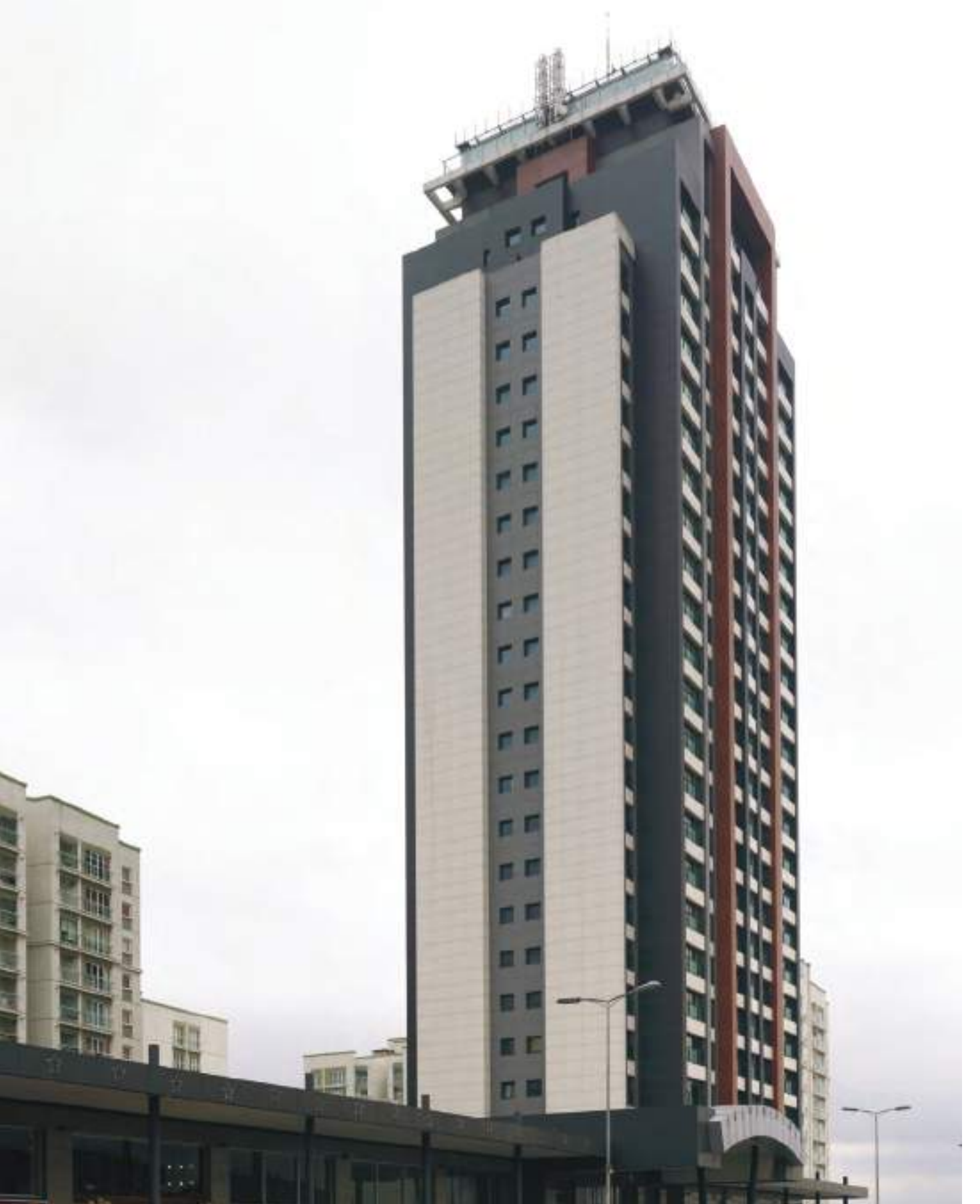
Avrupa Konutları / İstanbul — Kalesinterflex 3mm Fit Mat Beyaz, 3mm Fit Mat Kızıl, 3mm Fit Mat Koyu Gri, 3mm Fit Mat Siyah / Gizli Klipsli Sistem Avrupa Residence / İstanbul — Kalesinterflex 3mm Fit Matte White, 3mm Fit Matte Coral, 3mm Fit Matte Dark Grey, 3mm Fit Matte Black / Hidden Clips Fitted Facade System Mimar: Tekeli-Sisa Mimarlık — Architect: Tekeli-Sisa Architects
