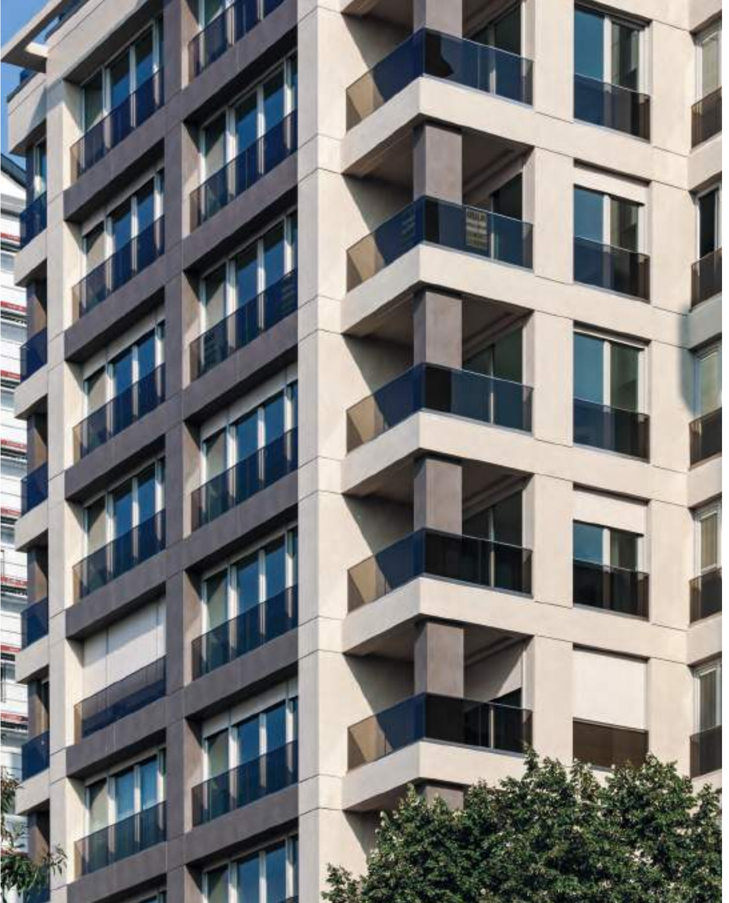
Ahenk Apartmanı Erenköy / İstanbul — Kalesinterflex 3mm Fit Leccese Grey, 3mm Fit Luxury Cement Vizon / Gizli Klipsli Sistem Ahenk Apartment Erenköy / İstanbul — Kalesinterflex 3mm Fit Leccese Grey, 3mm Fit Luxury Cement Mink / Hidden Clips Fitted Facade System Tavukçuoğlu İnşaat
