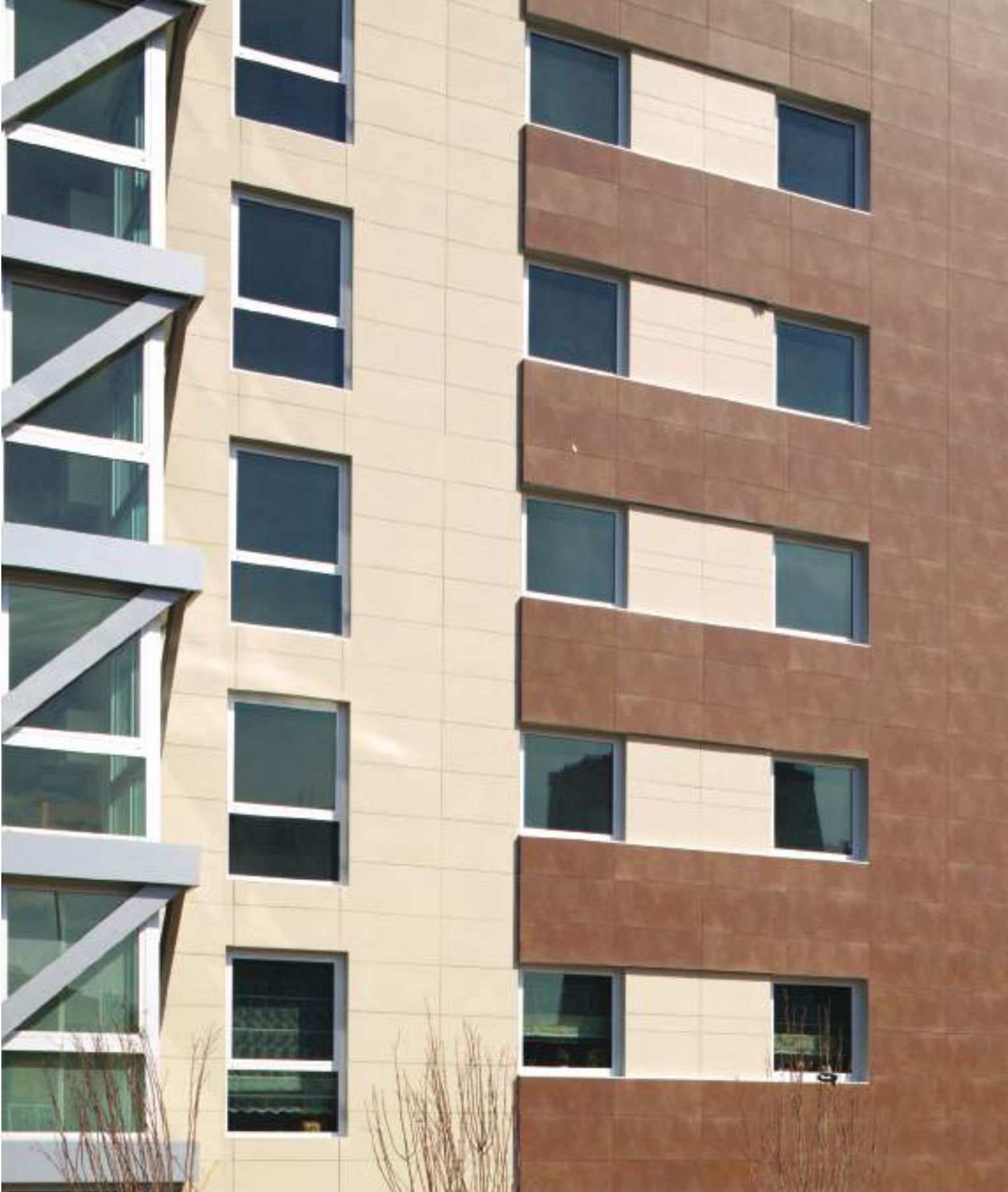
Mesa Park Oran Konutları / Ankara — 60x120cm Luxury Cement Kahve, 60x120cm Düz Bej Mat / Gizli Sistem Mesa Park Oran Residence / Ankara — 24"x48" Luxury Cement Brown, 24"x48" Solid Beige Matte / Invisible System Mimar: ACE Mimarlık — Architect: ACE Architectural Office
