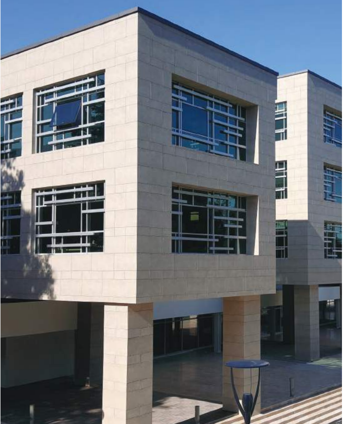
Bursa Teknik Üniversitesi / Bursa — 60x120 Cement 2.0 Kil Kaya Yüzey Bursa Technical University / Bursa — 60x120 Cement 2.0 Clay Rock Surface Mimar: Piray Mimarlık — Architect: Piray Architects
