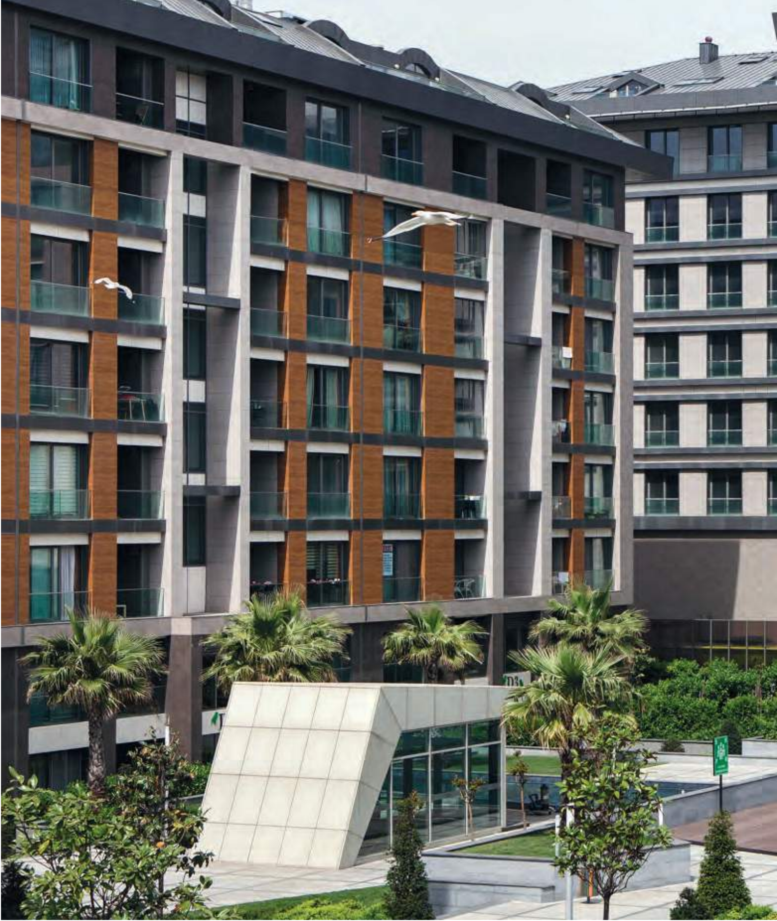
Ekşinar Konakları, Florya / İstanbul — 60x120cm Heraklia Stone Beyaz, Heraklia Stone Gri, Heraklia Stone Koyu Gri / Klipsli Sistem Ekşinar Residence, Florya / İstanbul — 24"x48" Heraklia Stone White, Heraklia Stone Grey, Heraklia Stone Dark Grey / Clips System Mimar: SPDO Mimarlık — Architect: SPDO Architectural
