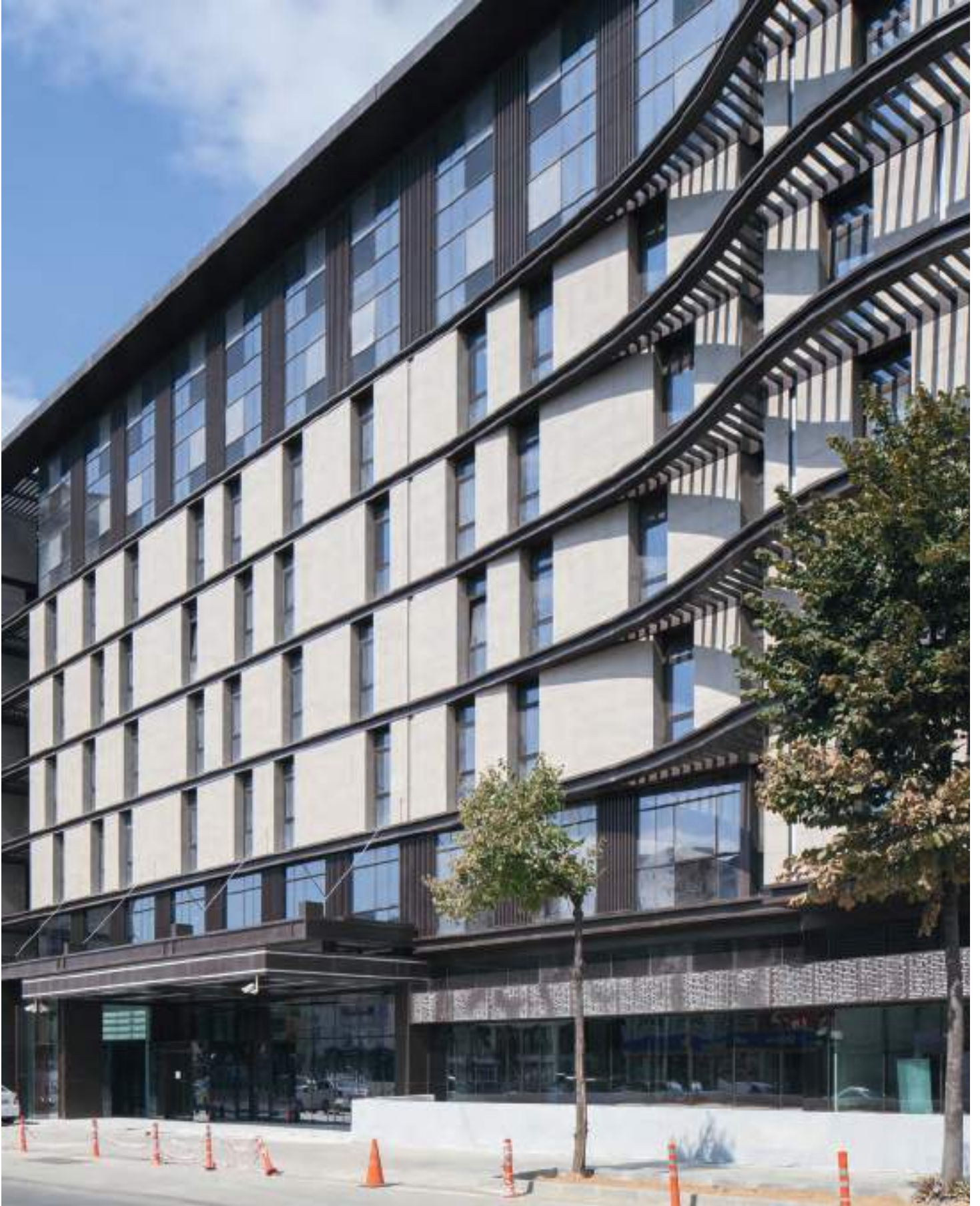
Burla Seba Otel, Dolapdere / İstanbul — 60x120cm / 60x60cm / 30x60cm Cement 2.0 Kil Mat / Konstrüksiyona Yapıştırma Sistem Burla Seba Otel, Dolapdere / İstanbul — 24"x48" / 24"x24" / 12"x24" Cement 2.0 Clay Matte / Adhesion System on Construction Mimar: Loft Mimarlık — Architect: Loft Architects
