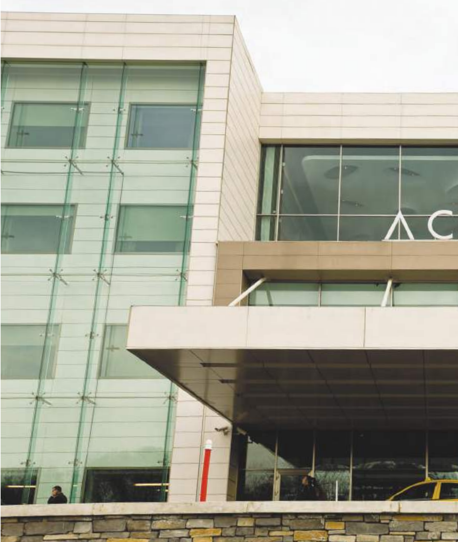
Acibadem Hastanesi, Maslak / İstanbul — Kalesinterflex 3mm Fit Mat Beyaz / Gizli Klipsli Sistem Acibadem Hospital, Maslak / İstanbul — Kalesinterflex 3mm Fit Matte White / Hidden Clips Fitted Facade System Mimar: Ertunga Mimarlık — Architect: Ertunga Architectural Office
