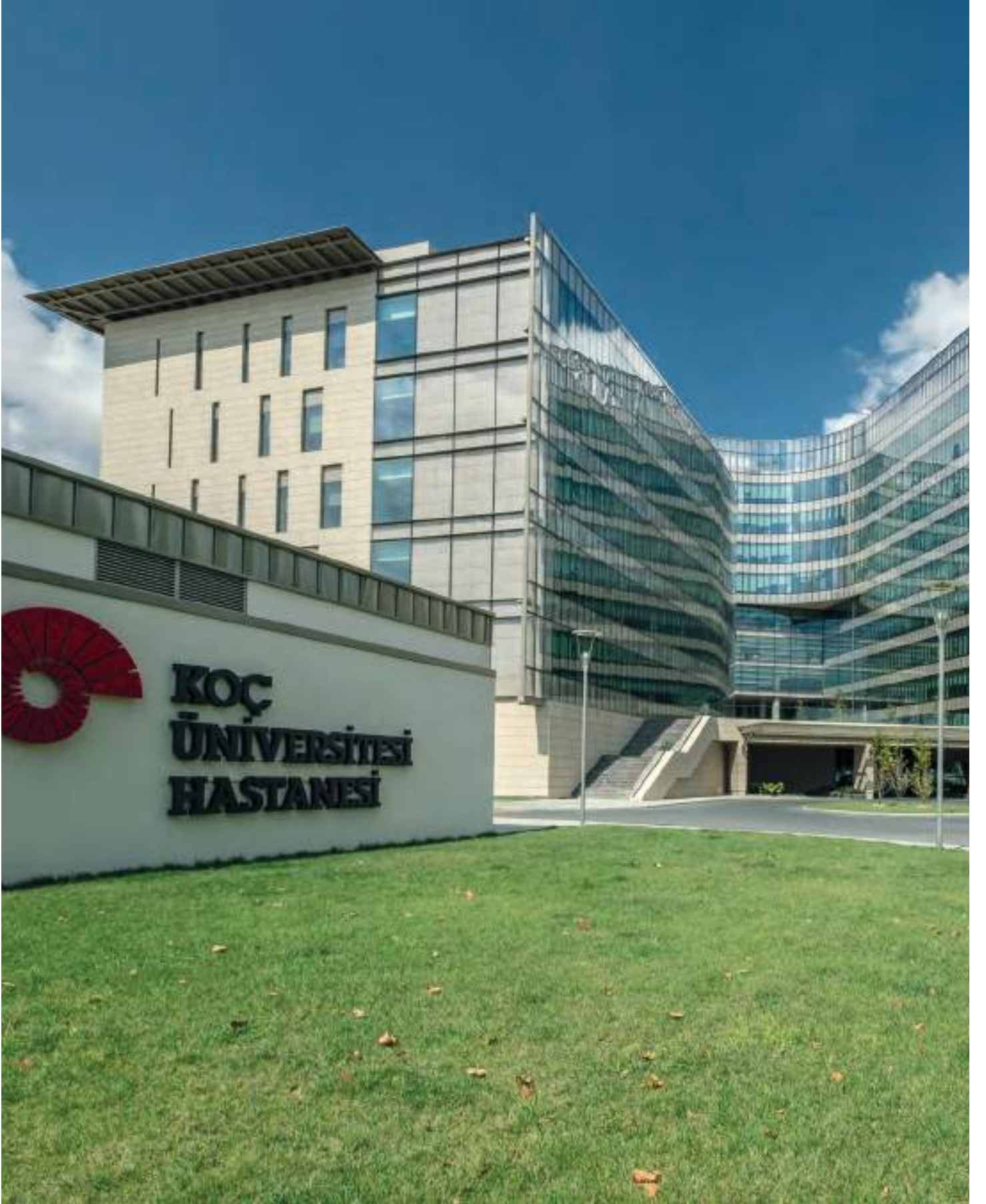
Koç Üniversitesi Tıp Fakültesi Hastanesi, Topkapı / İstanbul — Kalesinterflex 3mm Fit Leccese Grey / Gizli Klipsli Sistem Koç University School of Medicine, Topkapı / İstanbul — Kalesinterflex 3mm Fit Leccese Grey / Hidden Clips Fitted Facade System Mimar: Kreatif Mimarlık — Architect: Kreatif Architectural Office
