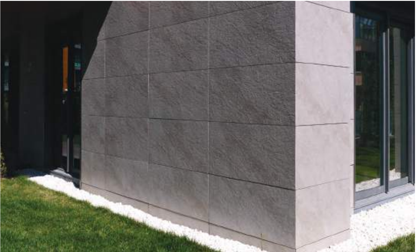
Avrupa Konakları, Florya / İstanbul — 60x120cm Heraklia Stone Gri / Gizli Sistem Avrupa Mansions, Florya / İstanbul — 24"x48" Heraklia Stone Grey / Invisible System Mimar: Sabri Paşayığıt Design Office — Architect: Sabri Paşayığıt Design Office
