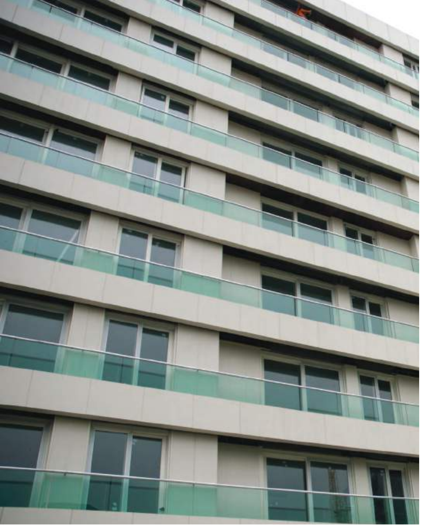
Novus Residence, Ataköy / İstanbul — Kalesinterflex 3mm Fit Mat Beyaz / Gizli Klipsli Sistem Novus Residence, Ataköy / İstanbul — Kalesinterflex 3mm Fit Matte White / Hidden Clips Fitted Facade System Mimar: TAGO Mimarlık — Architect: TAGO Architectural Office
