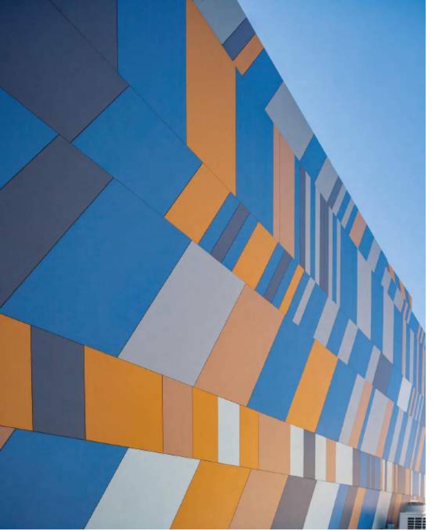
İRME Elektrik / İZMİR – Kalesinterflex 5mm Fit Mat Mavi, 5mm Fit Mat Turuncu, 5mm Fit Mat Safran, 5mm Fit Mat Çakıl Gri, 5mm Fit Mat Koyu Gri / Konstrüksiyon Üzeri Yapıştırma Sistem İRME Electric / İZMİR – Kalesinterflex 5mm Fit Matte Blue, 5mm Fit Matte Orange, 5mm Fit Matte Saffron, 5mm Fit Matte Pebble Grey, 5mm Fit Matte Dark Grey / Adhesion System on Construction Mimar: Arda Işık Mimarlık — Architect: Arda Işık Architects
