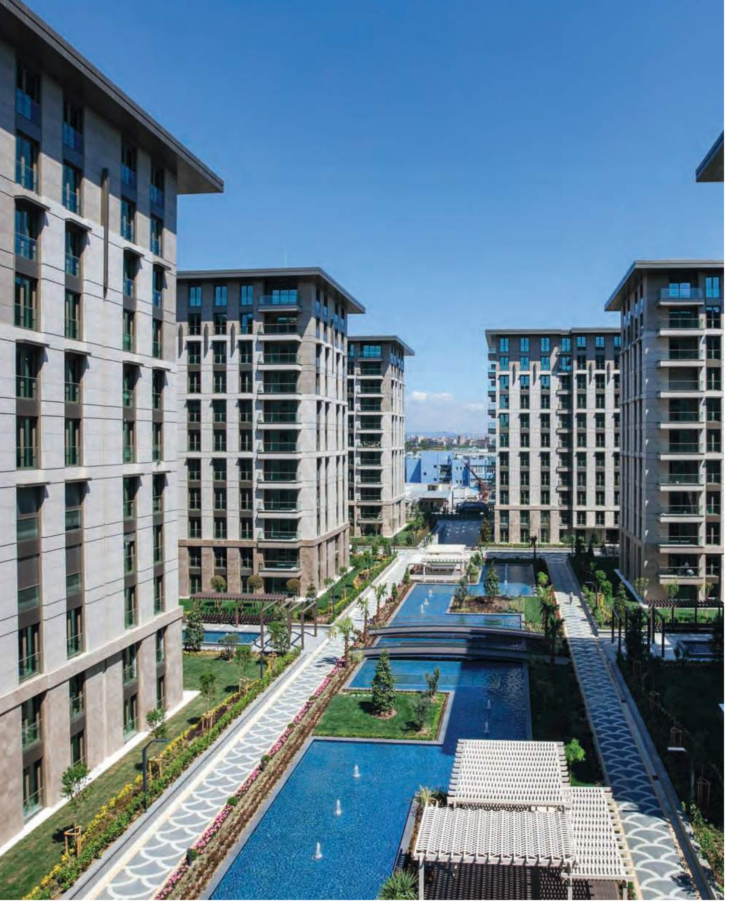
Avrupa Konutları, Topkapı / İstanbul — Kalesinterflex 3mm Fit Limestone, 3mm Fit Sandstone GY305 / Gizli Klipsli Sistem Avrupa Residence, Topkapı / İstanbul — Kalesinterflex 3mm Fit Limestone, 3mm Fit Sandstone GY305 / Hidden Clips Fitted Facade System Mimar: Viva Mimarlık — Architect: Viva Architects
