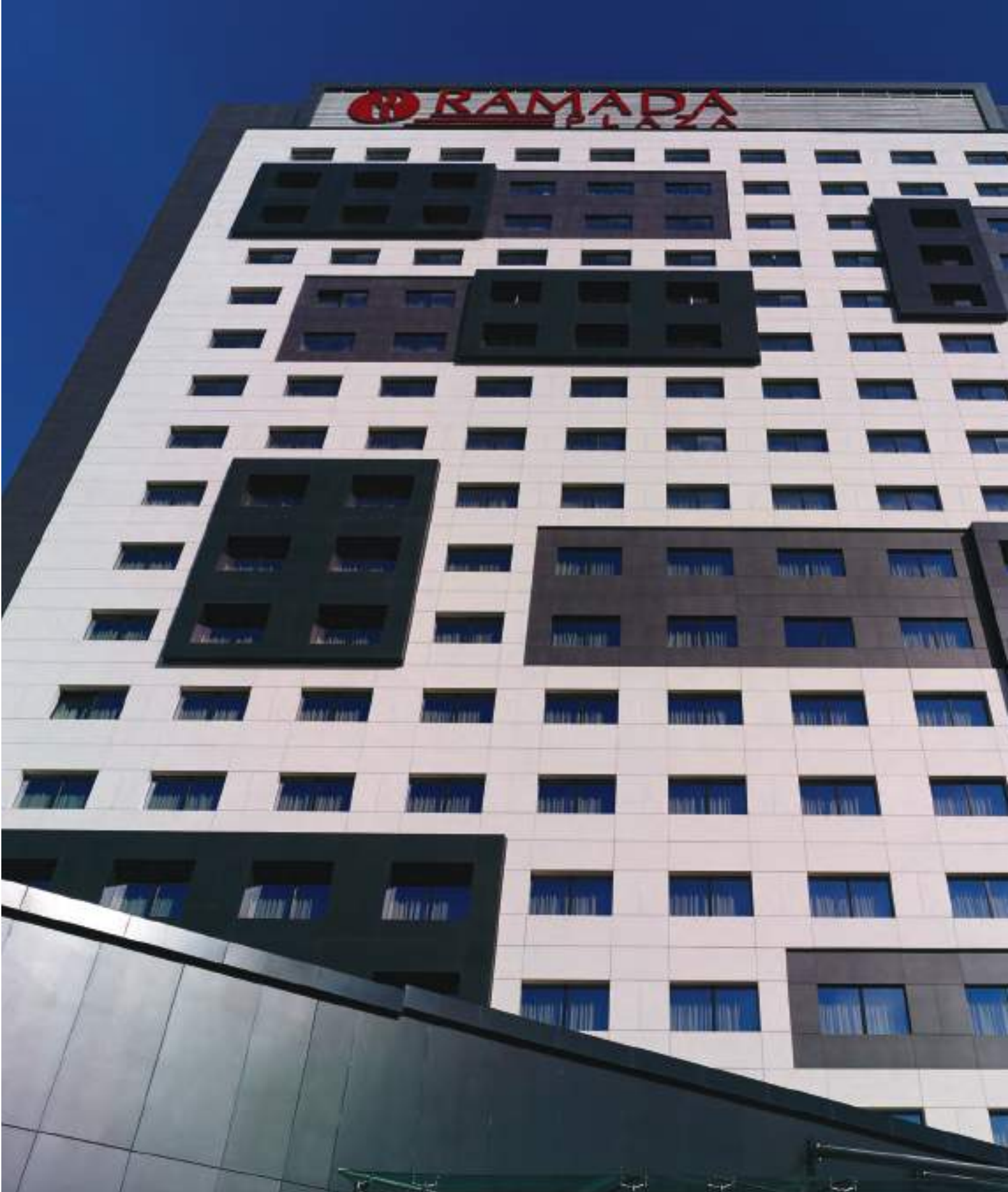
Ramada Plaza / İstanbul — Kalesinterflex 3mm Fit Mat Mega Siyah, 3mm Fit Mat Mega Beyaz, 3mm Fit Luxury Cement Antrasit / Gizli Klipsli Sistem Ramada Plaza / İstanbul — Kalesinterflex 3mm Fit Matte Mega Black, 3mm Fit Matte Mega White, 3mm Fit Luxury Cement Anthracite / Hidden Clips Fitted Facade System Mimar: M Ofis — Architect: M Office
